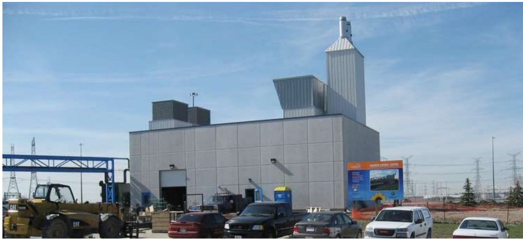
The Markham District Energy System will have four locations when completed. Photo left – Construction nears completion on the second site in April 2008.
