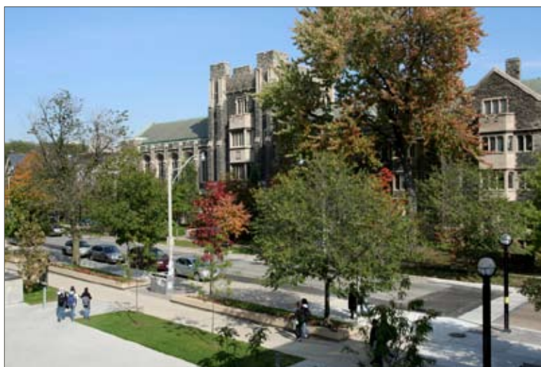
The University of Toronto's St. George Campus is served by a combined heat and power system that can provide six megawatts of electricity to the campus. The Medical Sciences Building (top) features two absorption chillers that uses system steam for cooling.
