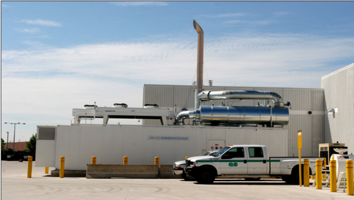
Left, 1.2 MW Go Transit CHP Plant with roof-mount heat exchange system; right, Go Transit Streetsville bus maintenance area.
