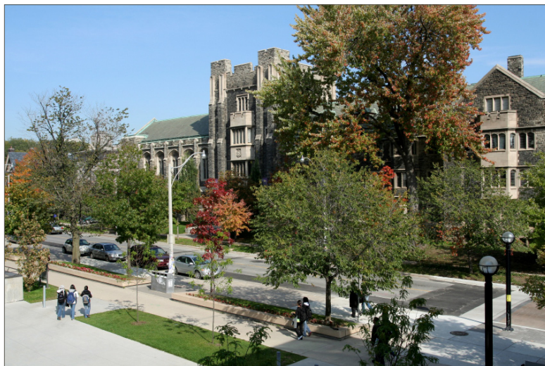
The University of Toronto's St. George Campus is served by a combined heat and power system that can provide six megawatts of electricity to the campus. The Medical Sciences Building (top) features two absorption chillers that use system steam for cooling.
