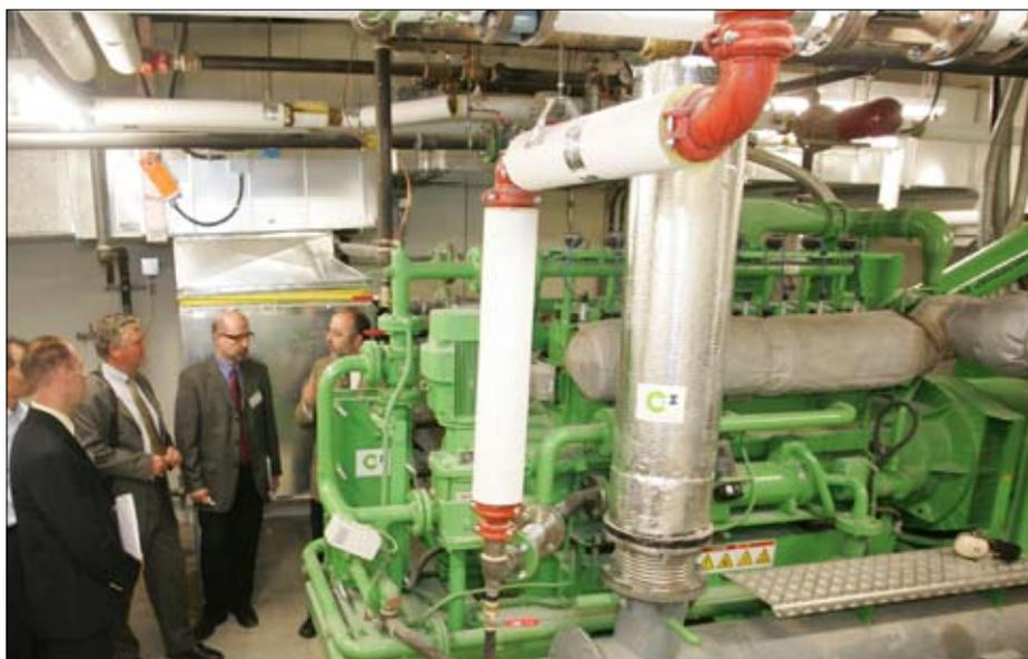
The natural gas cogen system in the Villa Colombo Vaughan provides emergency power, electricity and hot water for both space heating and domestic hot water supplies.
