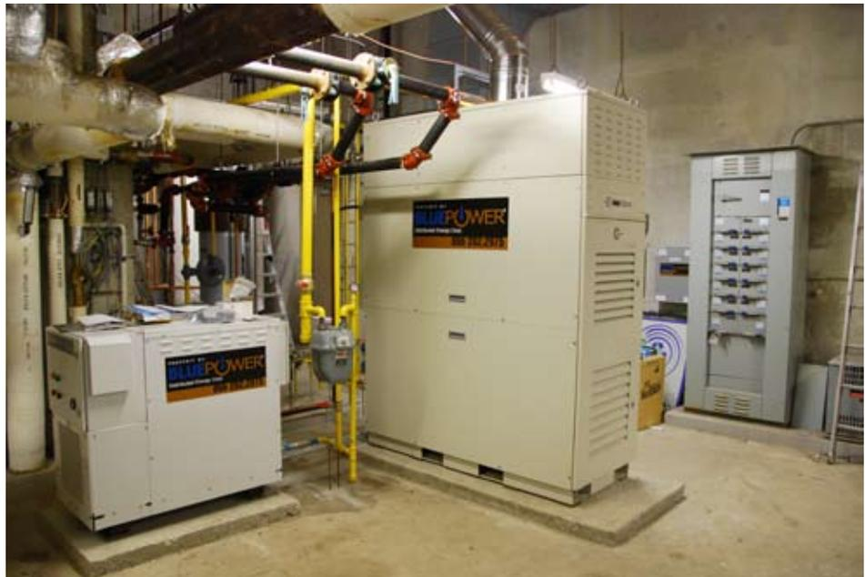
The Capstone turbine system installed at the Aurora Green Condominium is a good alternative to a conventional boiler. And because the modular system can be easily expanded, it is also a good way to get started with a CHP system.
